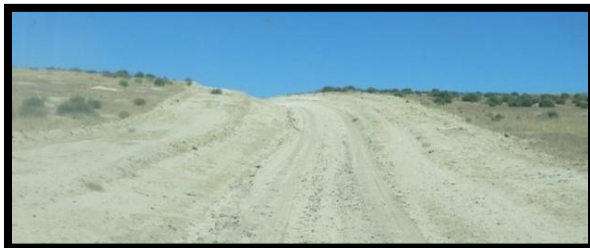
The road was graded on both sides to serve as a firebreak
