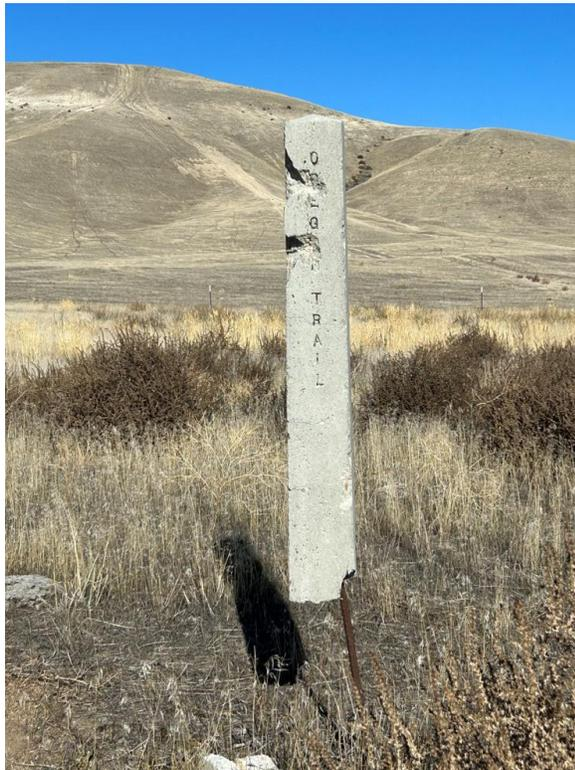
Concrete Oregon Trail marker has been badly damaged by gunshots. Note it is still standing on the rebar running up the center of the post. Photo by Paul Dinwiddie
