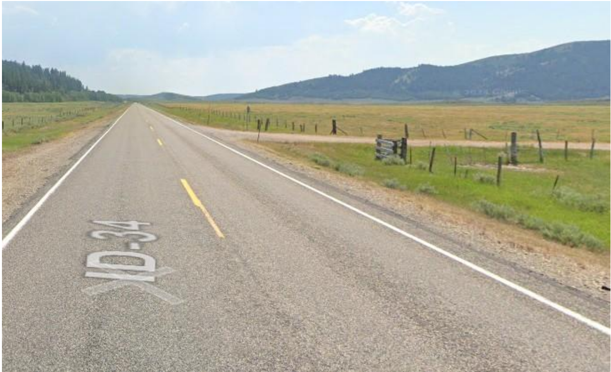
PHOTO K (WAYPOINT 26) Looking South
